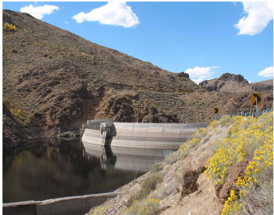
Photo 5.10. Wild Horse Reservoir is impounded behind a double-curvature arch dam completed in 1969 to replace the original dam, Nevada
