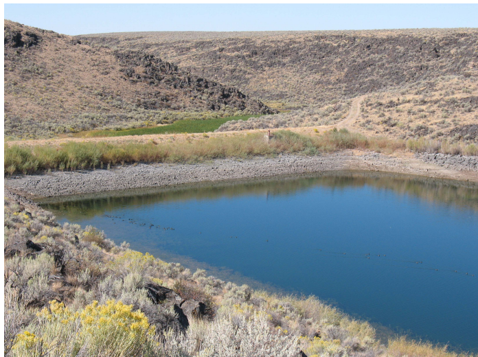
Photo 5.1. Wilson Reservoir dam, Nevada
