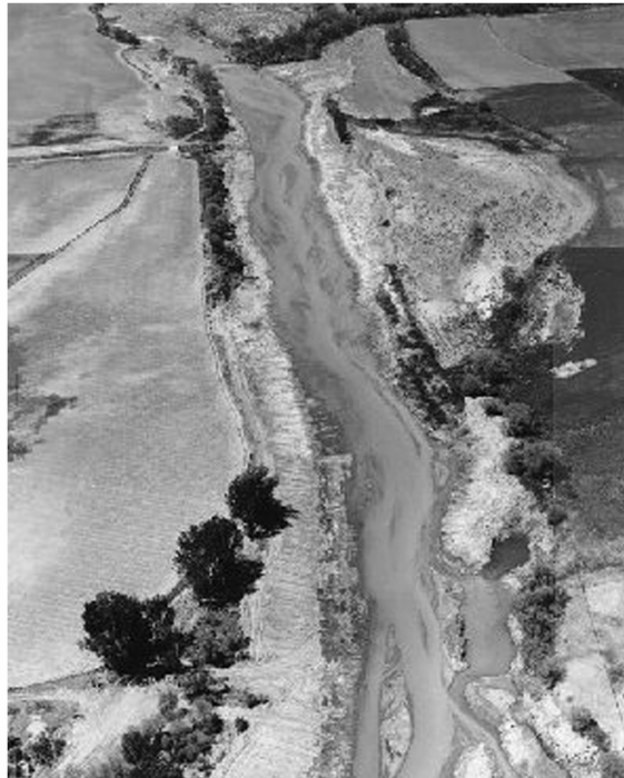
Figure 12.1. Army Corps of Engineers clearing and snagging of the Owyhee River below Owyhee Dam, 1954.
